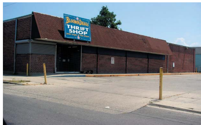
Existing Freret Street Building
